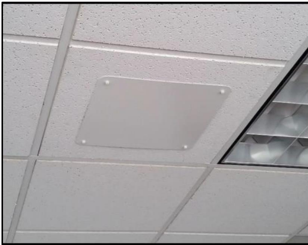
Installed Antenna
