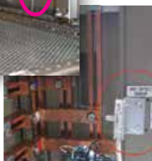
Examples of Arc-Flash Relay light sensor installation in switchgear.
