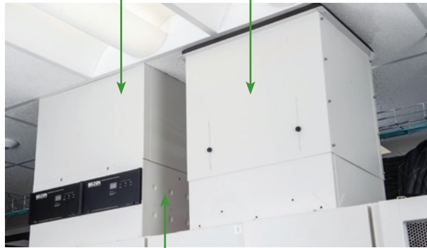
Example of passive and active chimney systems
