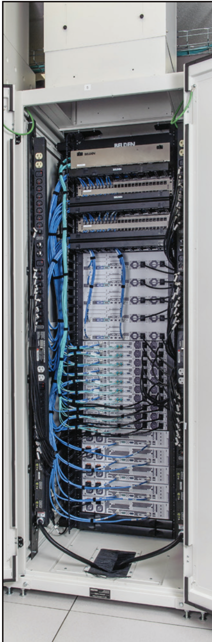
Organized networking and power cable management for proper server airflow
